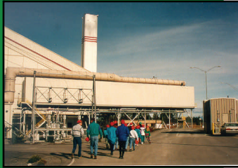
Learn where your garbage goes with a tour of Spokane's Waste to Energy Plant
